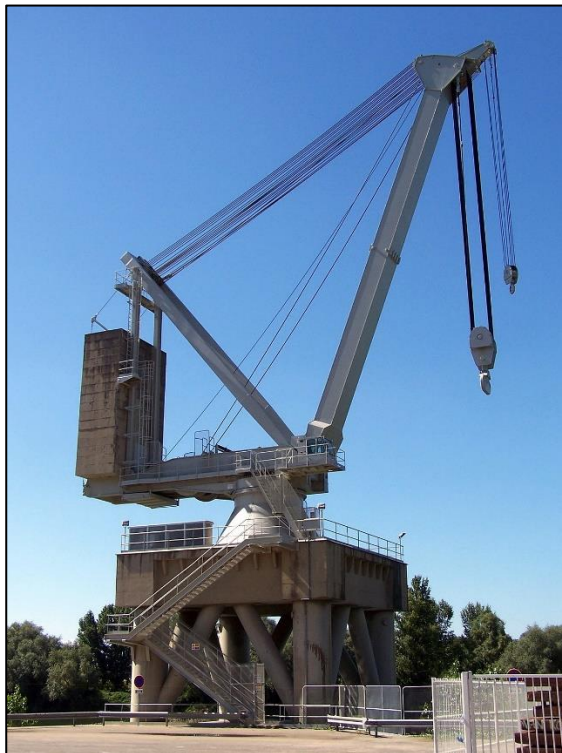
Figure 20 : Grue fixe EDF.
