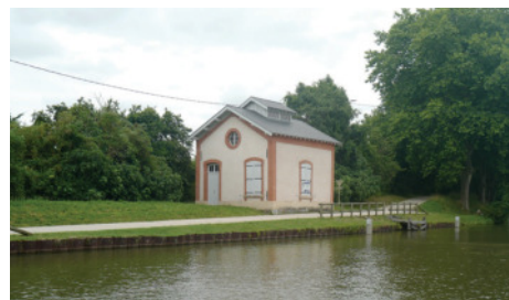
[ancienne station de pompage, Montgiscard]
