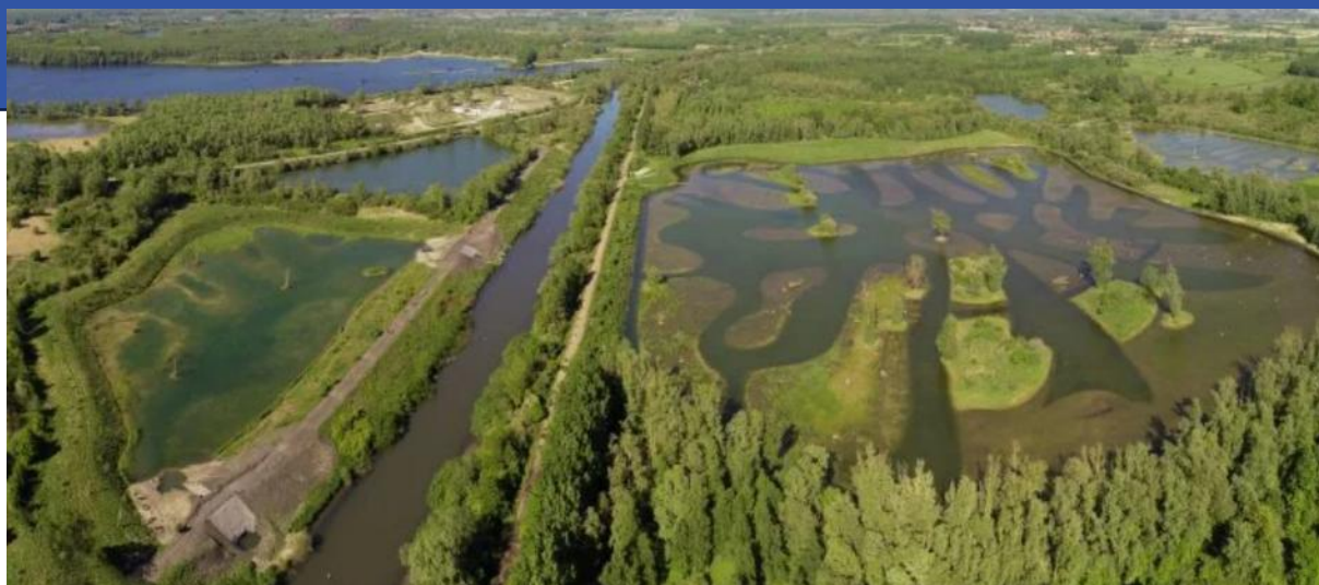
© VNF Houzé – Grand Marais de la Fosse Saint Pierre (59)
